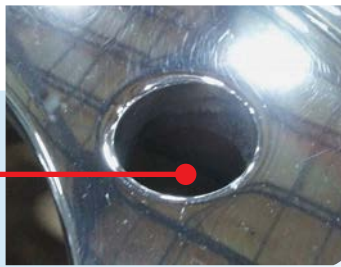
BOLT HOLE WASHOUT
